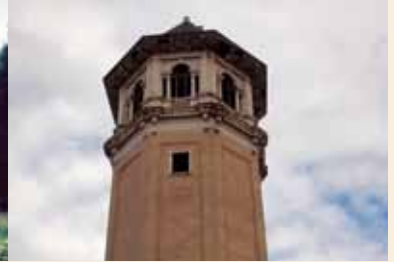
THE ROLAND WATER TOWER
