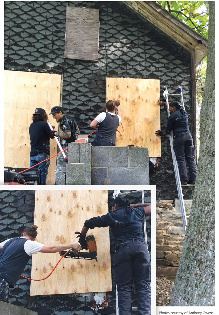
Photos courtesy of Anthony Owens Remodeling and Repair
