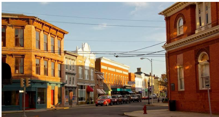
In Cambridge, 11 Poplar Street was restored with the Sustainable Communities Tax Credit. The total private investment was $225,000 and created 3 jobs, with a tax credit amount of $45,000.
