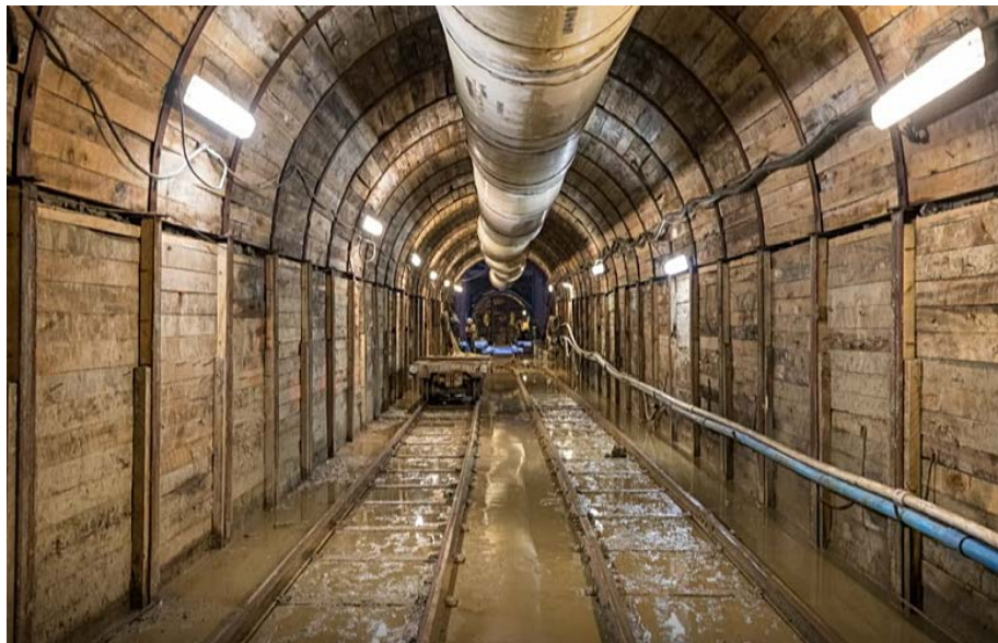
Figure 1. 19 th century underground tunnels that manage stormwater in Charleston.
