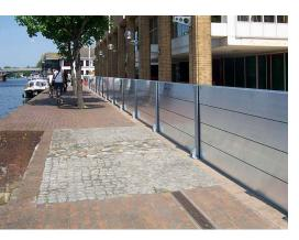
Demountable Flood Barriers can be retrospectively fitted to suitable existing foundations
