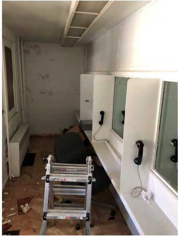
Photo 6: ACM Positive W-17 and W-18, Orange vinyl floor tile and mastic.
