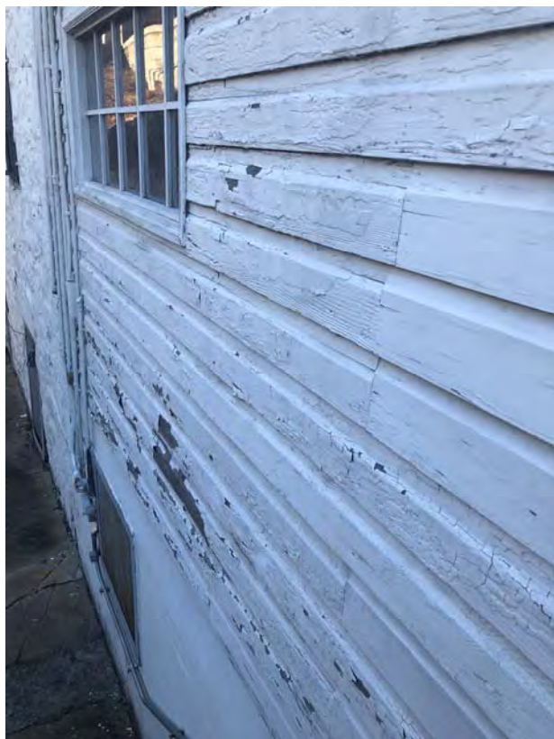
Photo 7: LBP Positive, White Exterior Wood Wall and Window.
