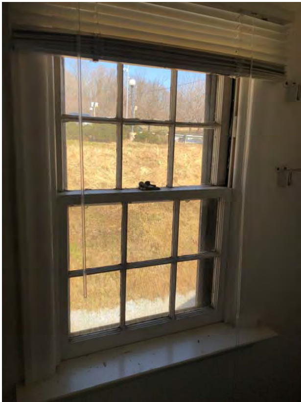
Photo 5: ACM Positive EA-30 and EA-34, Beige Window Caulk and White Window Glaze with Double Hung Windows.
