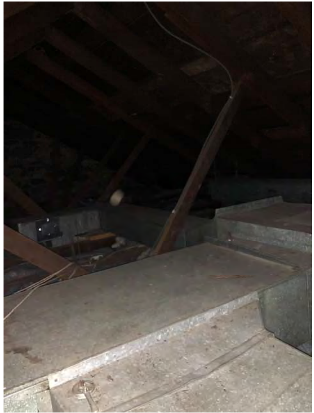
Attic, evidence of water intrusion and visible mold growth.
