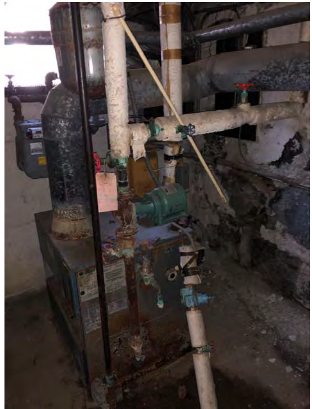
Room 26, evidence of water intrusion and visible mold growth.
