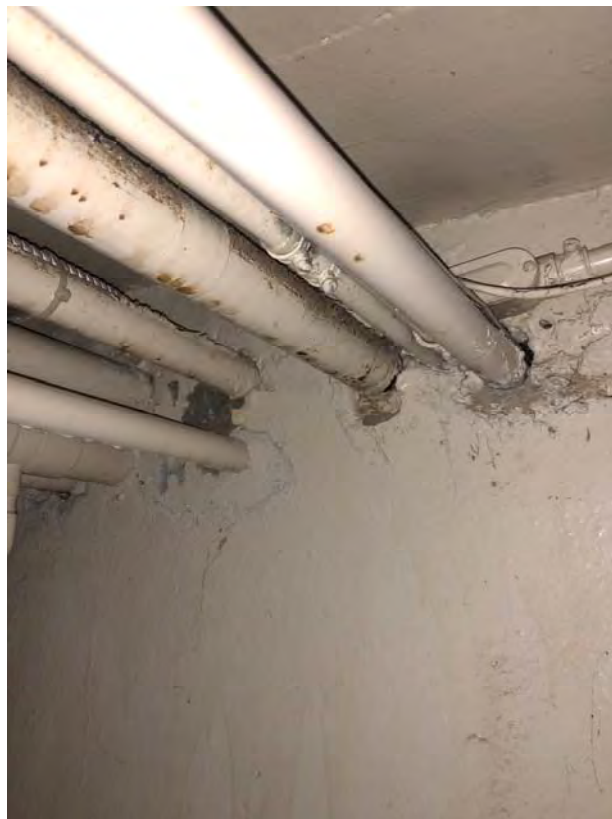
Photo 4: ACM Positive EA-27, Yellow Pipe Penetration Caulk/Foam
