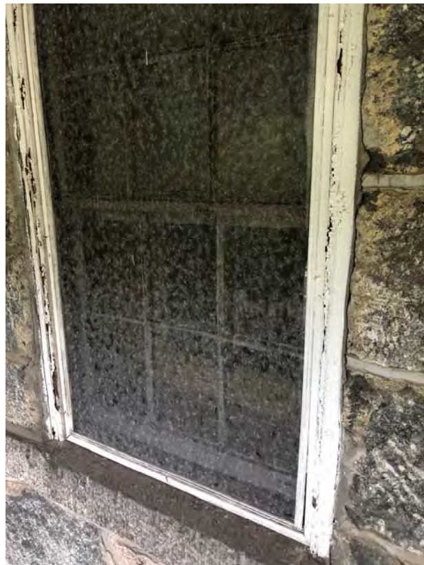
Photo 44: LBP Positive, White Wood Window Frame/ Casing.
