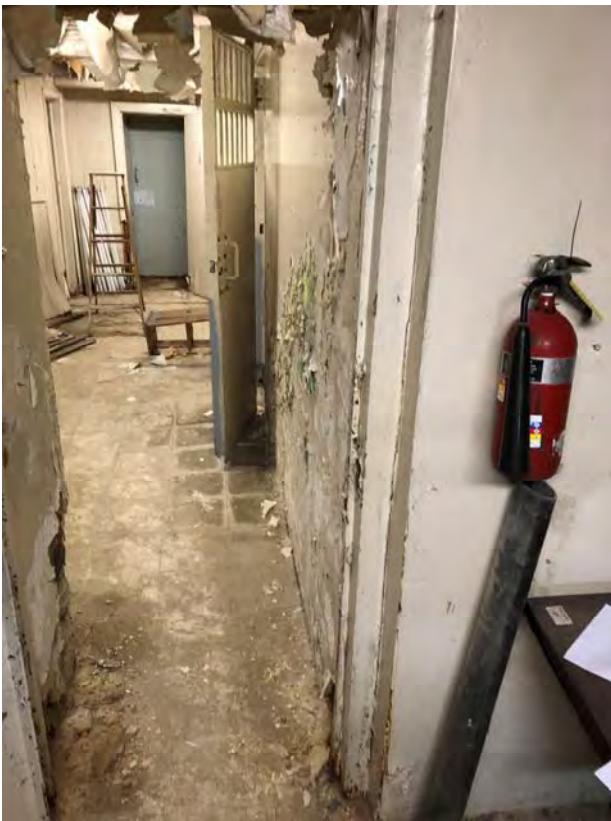
Photo 29: LBP Positive, Brown Masonry Wall.
