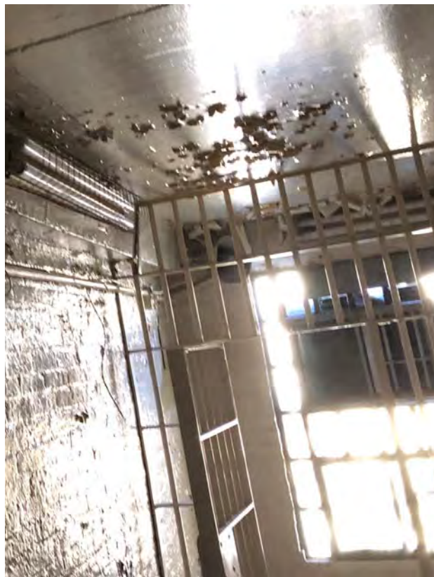
Photo 2: ACM Positive EA-24, White Window Caulk Associated with Metal Fold-in Windows. LBP Positive, White Window Guard.
