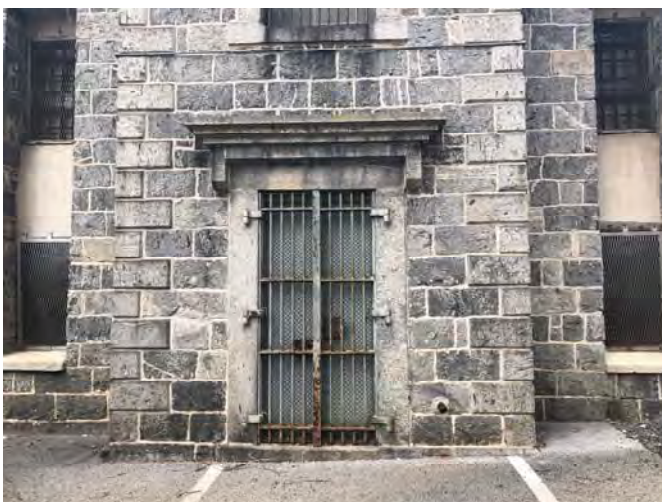
Photo 11: LBP Positive, Exterior Metal Door.
