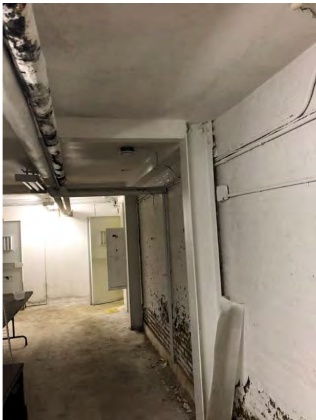
Photo 37: LBP Positive, White Concrete Ceiling, White Masonry Wall, and White Metal Structural Beam.
