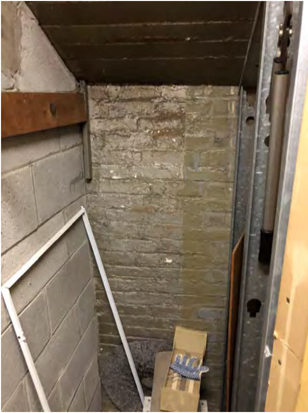
Photo 29: LBP Positive, Brown Masonry Wall.
