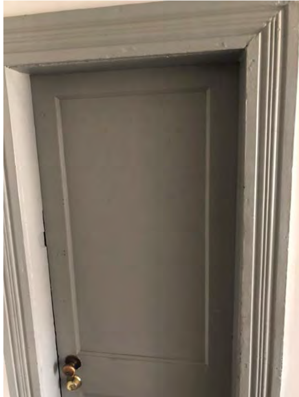
Photo 13: LBP Positive, Gray Decorative Wood Door Frame/Casing.
