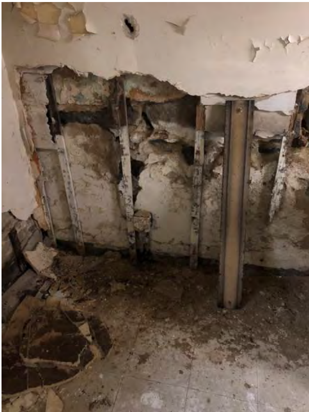
Room 28, wall damaged due to water intrusion and visible mold growth on building components.
