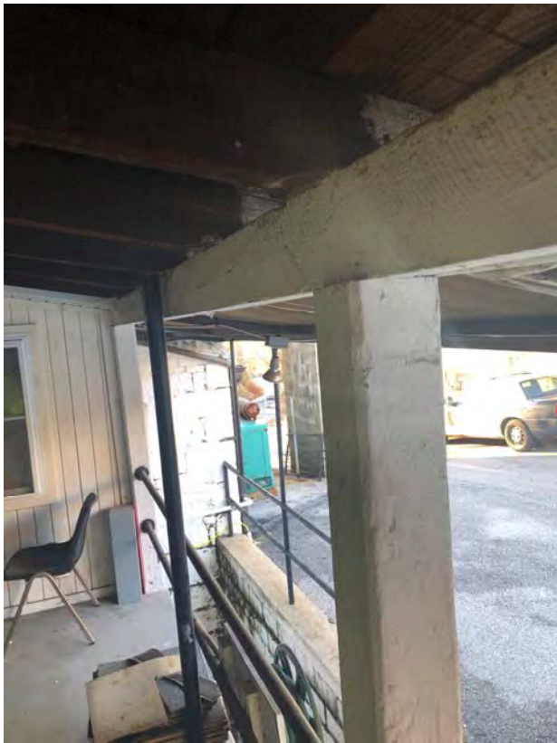
Photo 12: LBP Positive, White Wood Structural Beam and White Wood Joist.
