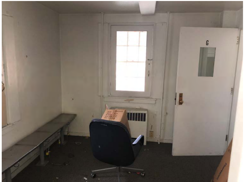
Photo 21: LBP Positive, White Metal Baseboard, White Metal Window, and White Wood Window Sill.
