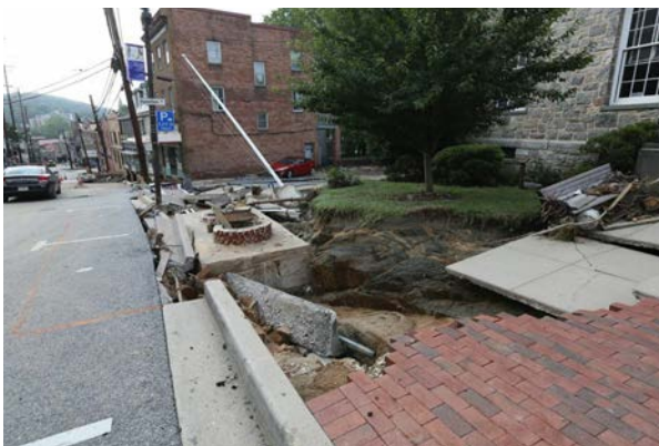
Figure 95: Damage to Brick Paving after the 2018 Flood
