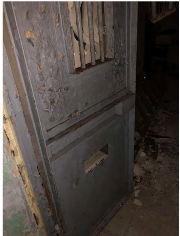
Photo 30: LBP Positive, White Metal Door Frame.
