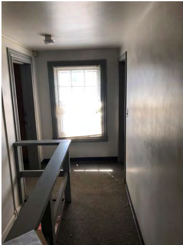
Photo 17: LBP Positive, Gray Decorative Wood Window Frame/Casing and White Drywall Ceiling.
