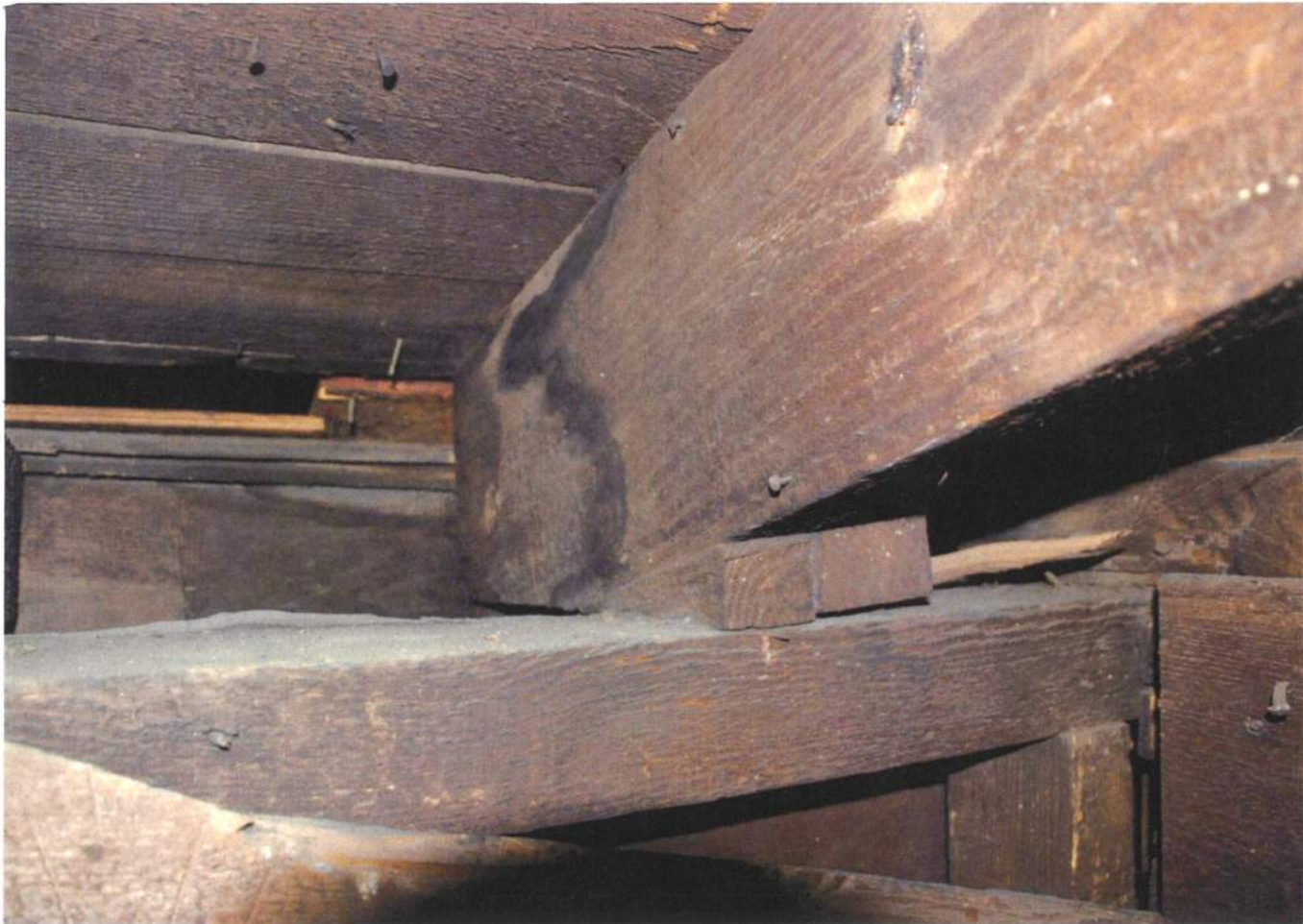
Attic framing at eave showing rafters and blocking. Looking southeast.
