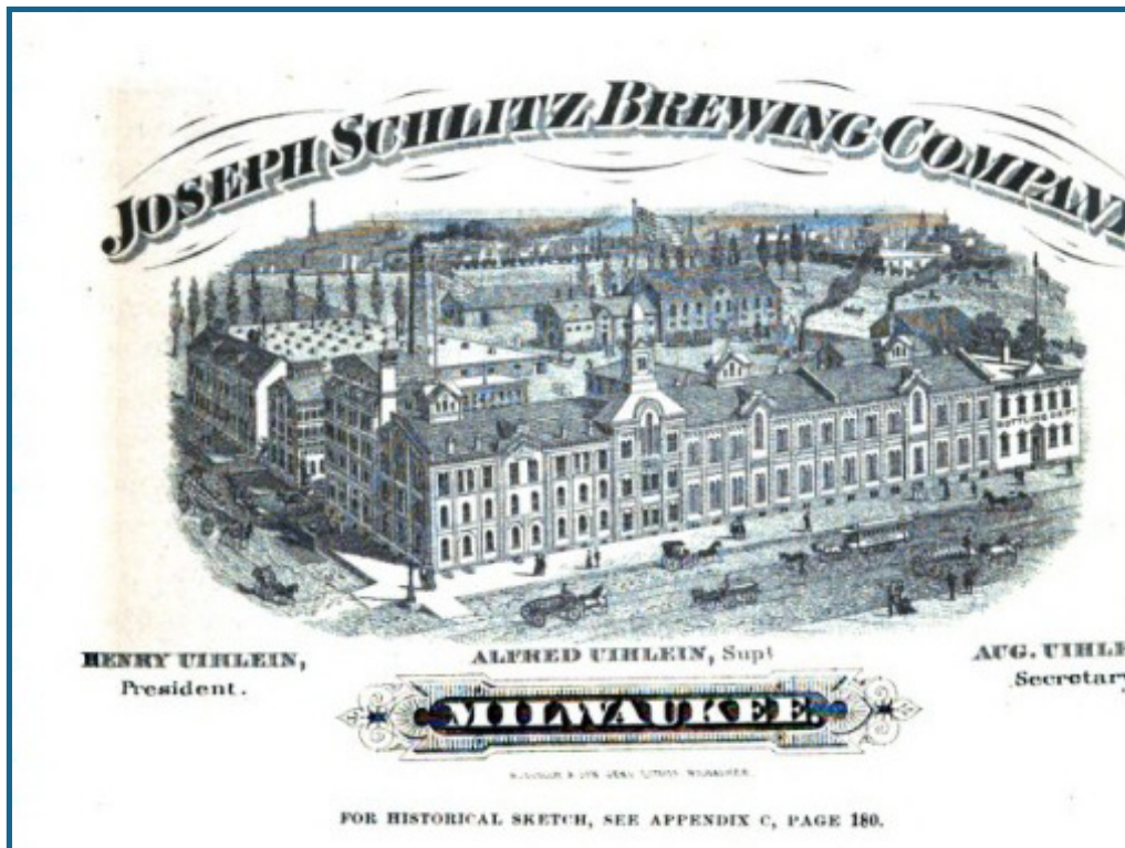
Figure 5.16 Schlitz Brewing Company, Milwaukee, Wisconsin (Source: Salem 1880)
