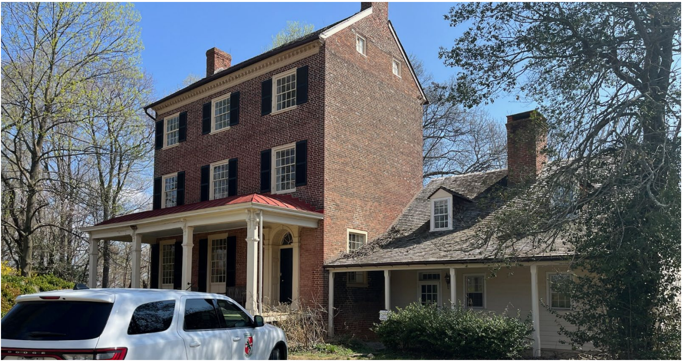
Front view (west elevation) of structure: 1½-story, mid-18th-century log house joined to 3-story, early-19th-century Federal-style brick wing
