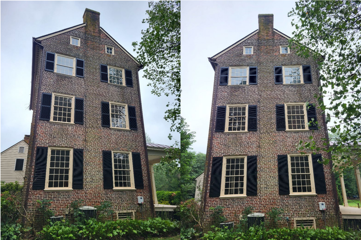
Side view (northern elevation) of the brick wing.
