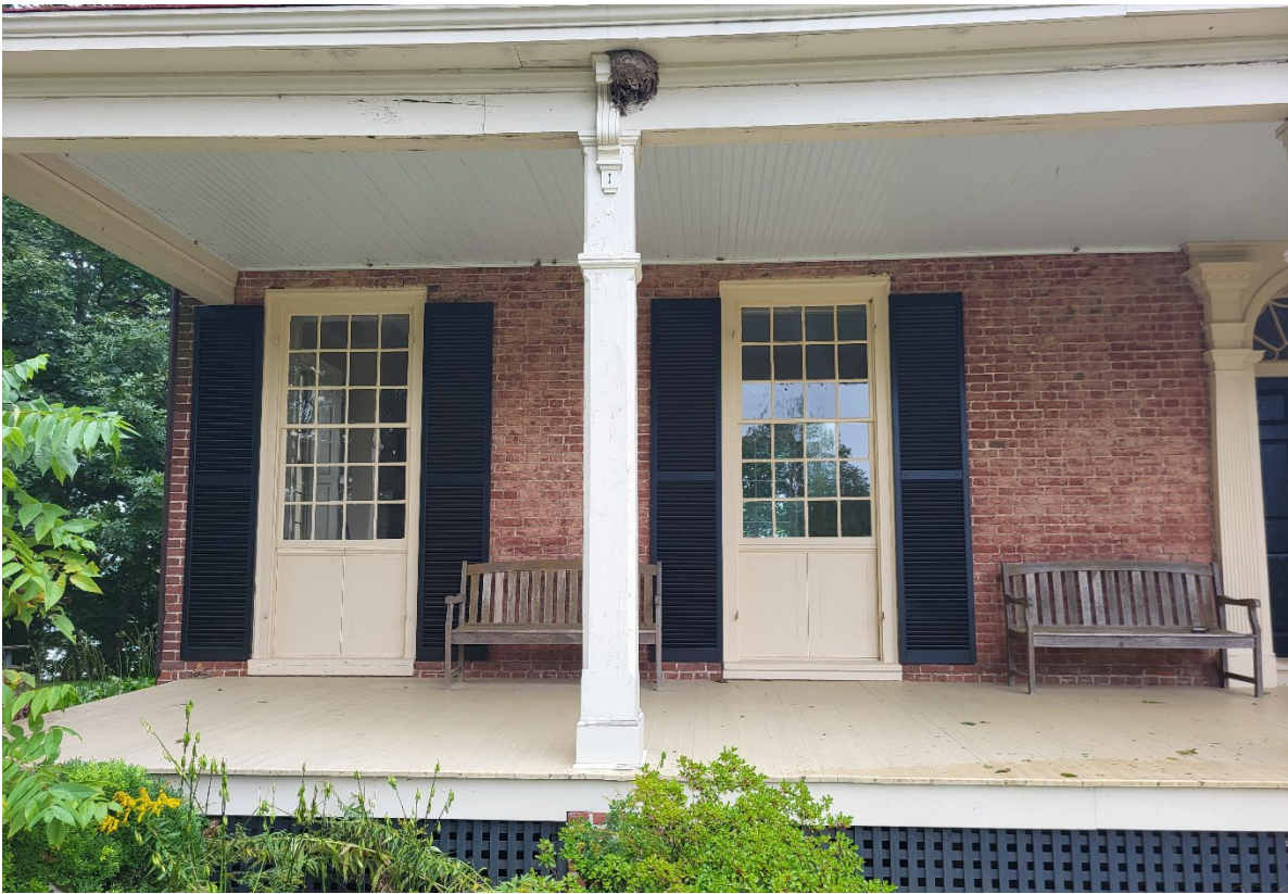
Main block porch with metal roof.
