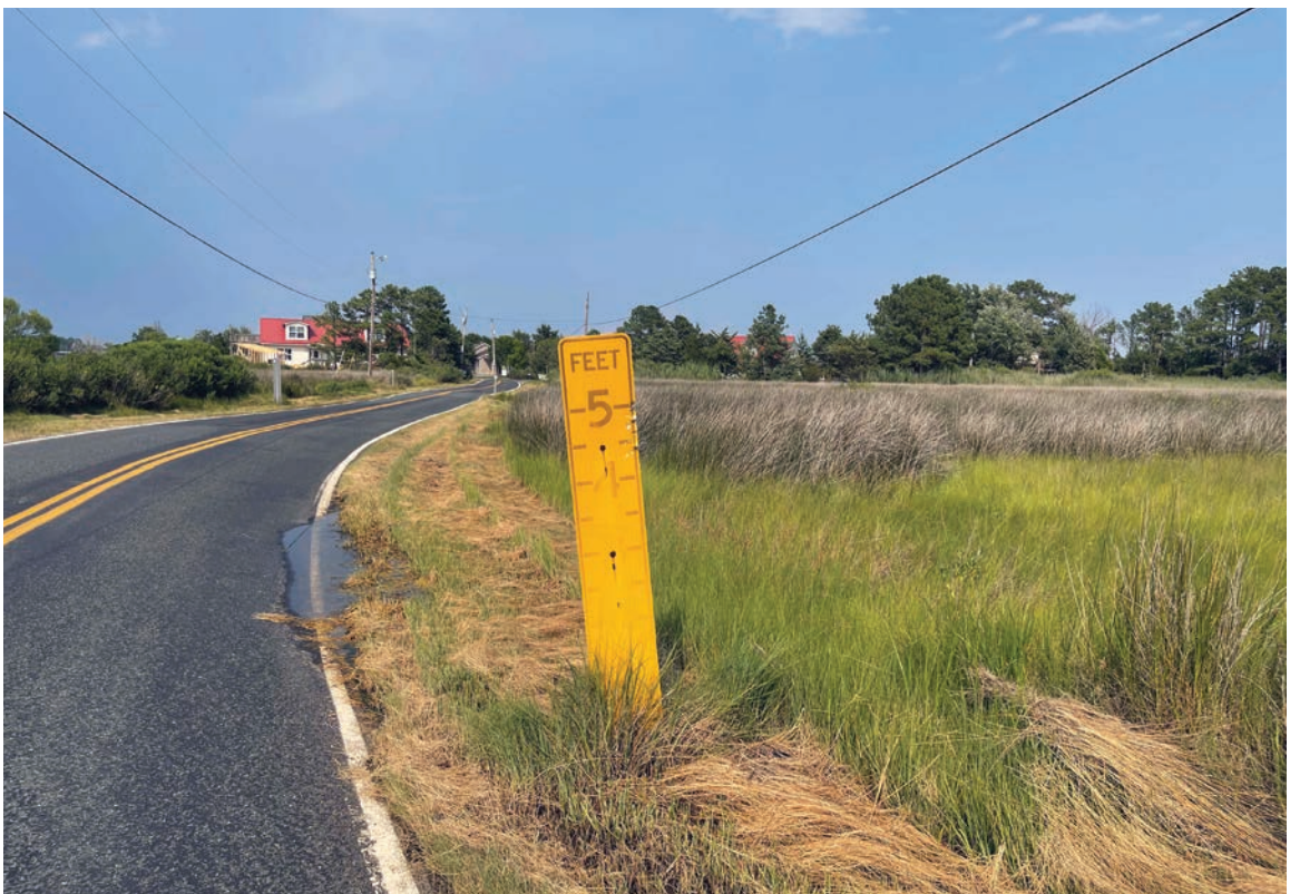
Figure 10.5: Sections of roads are flanked by water and are subject to flooding.
