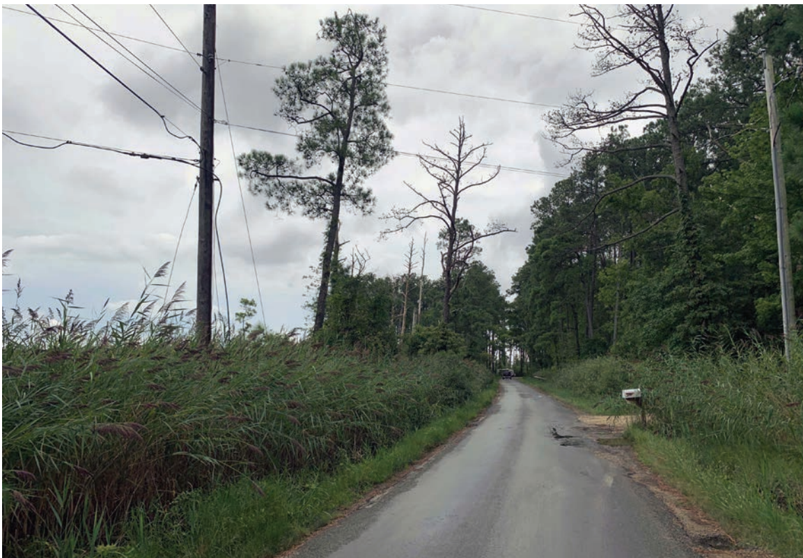
Figure 10.3: Some sections of the roadways have very narrow shoulders or do not have shoulders.
