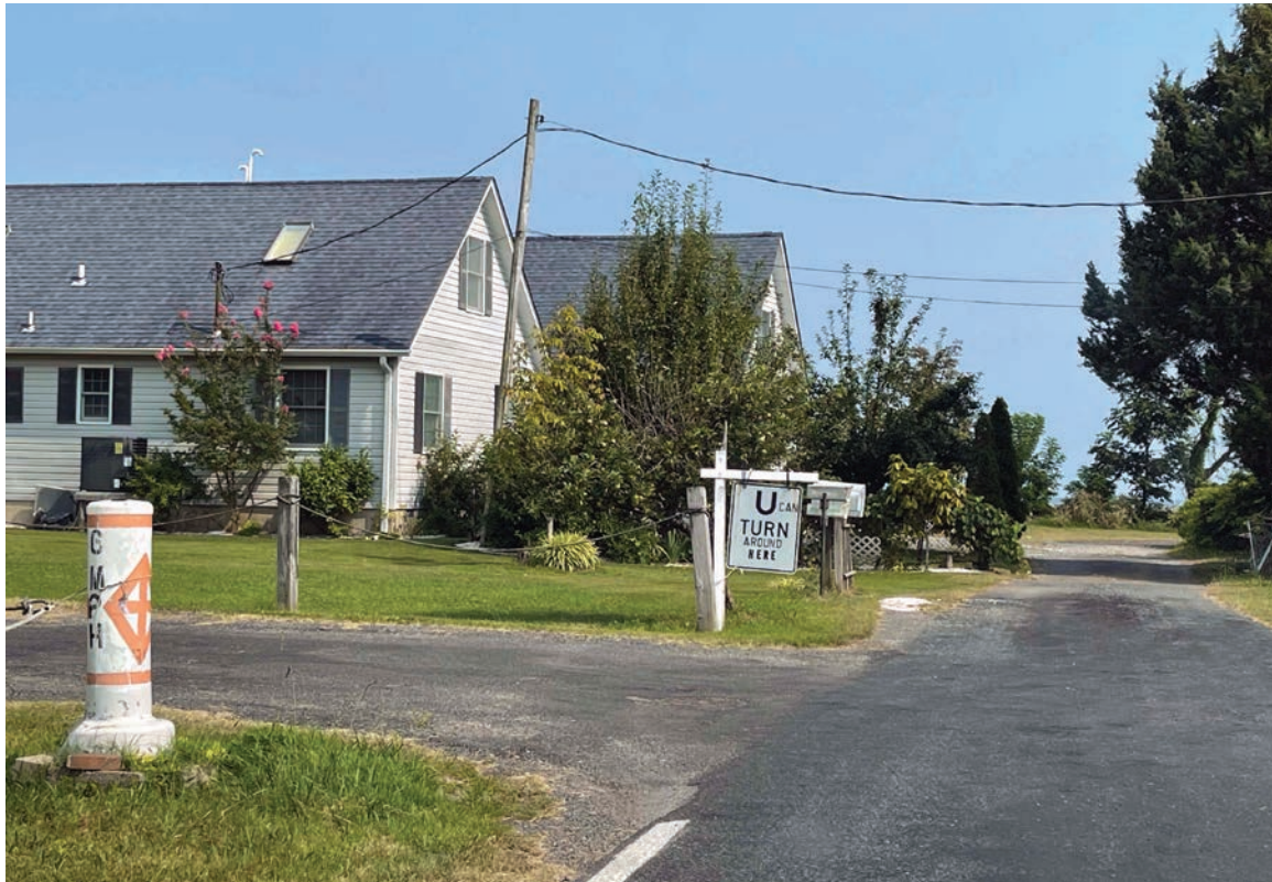
Figure 10.6: Many roads are terminated with private drives requiring access to these private drives to turnaround vehicles.
