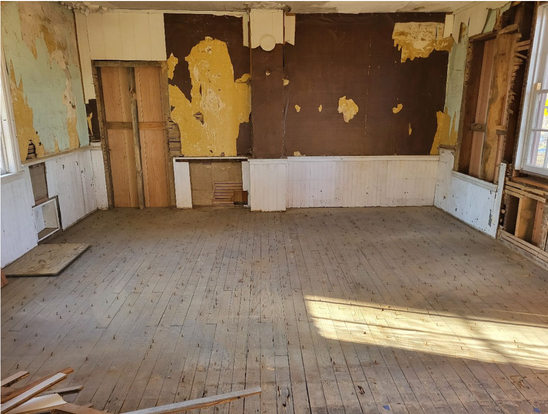
Back of Schoolhouse (West Interior)
