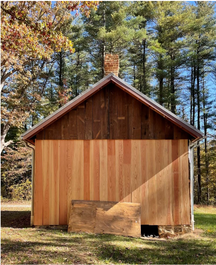
Back of Schoolhouse (West Exterior)
