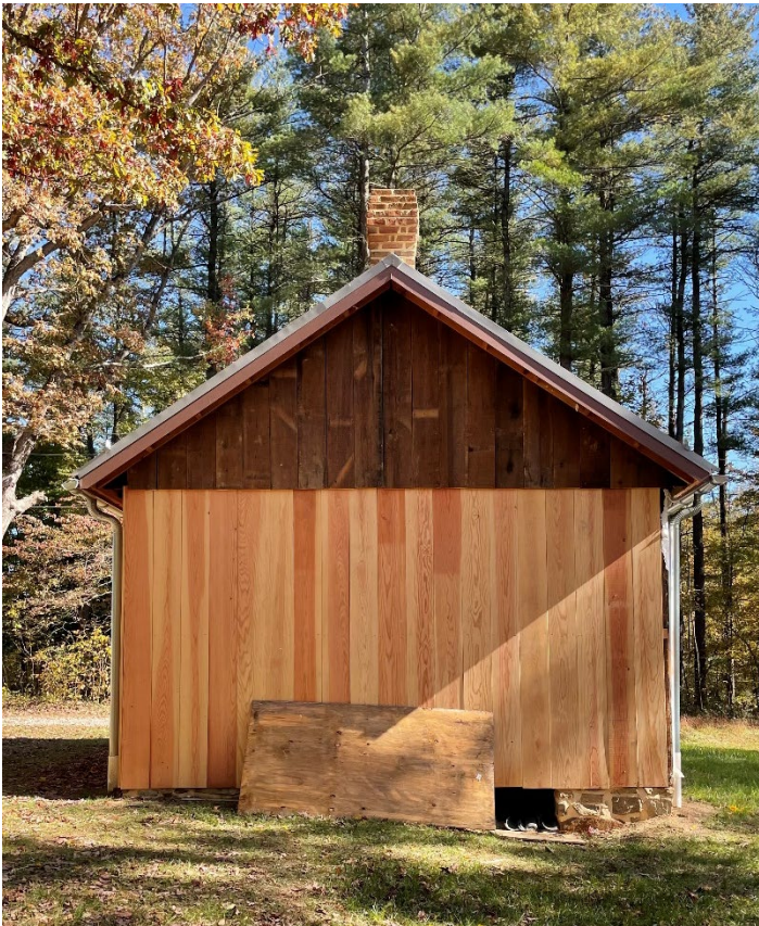
Back of Schoolhouse (West Exterior)
