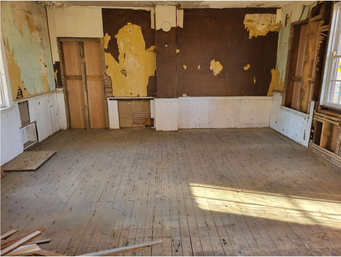
Back of Schoolhouse (West Interior)
