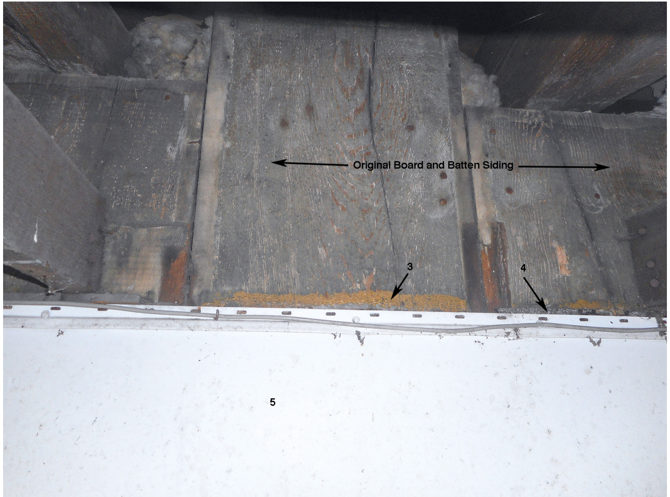
Illustration 2: North elevation, looking above the porch ceiling
