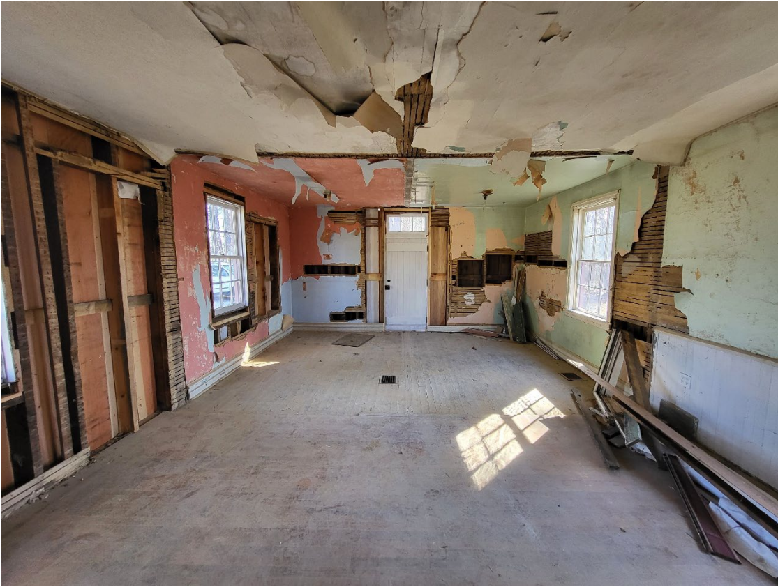
Front of Schoolhouse (East Interior)
