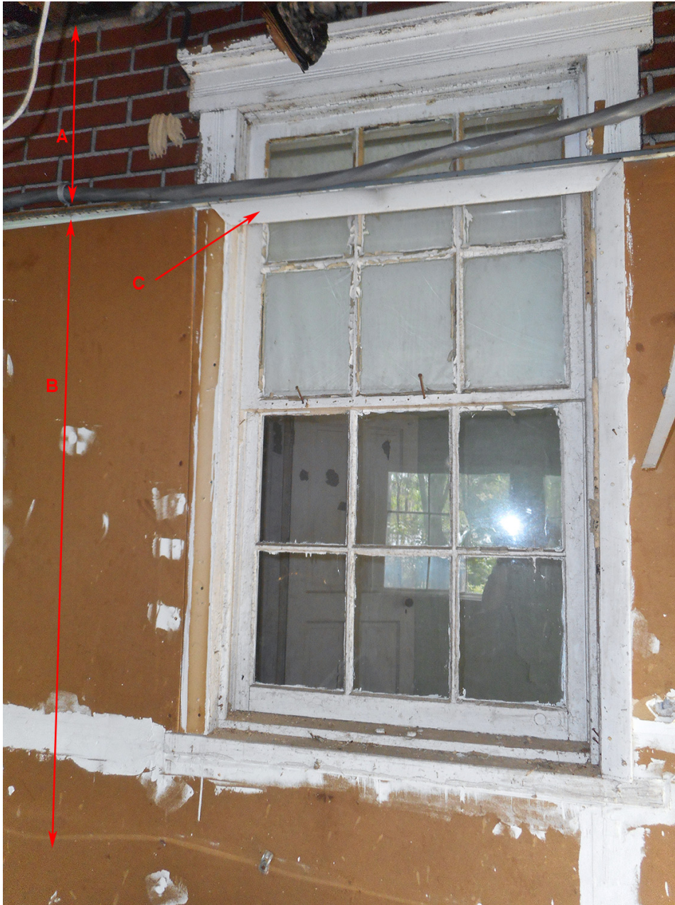
Site photograph: South Elevation post 1914 asbestos siding and later changes.
